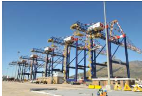
With a total of six new Liebherr ship-to-shore cranes in place, Berth 601 offers high productivity container handling.
